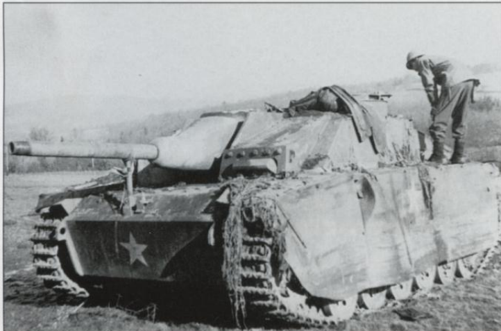
Besides the Panther tanks, five StuG III assault guns were converted for Panzer Brigade 150. Since they bore no resemblance at all to any US vehicle, their camouflage seems rather odd. The muzzle brake was removed, and side skirts added. This one was abandoned near the Baugnez crossroads, site of the infamous Malmédy massacre.
